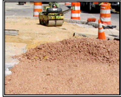
Structural Soils (from “Tree Space Design” produced by Casey Trees, in Washington D.C.)
